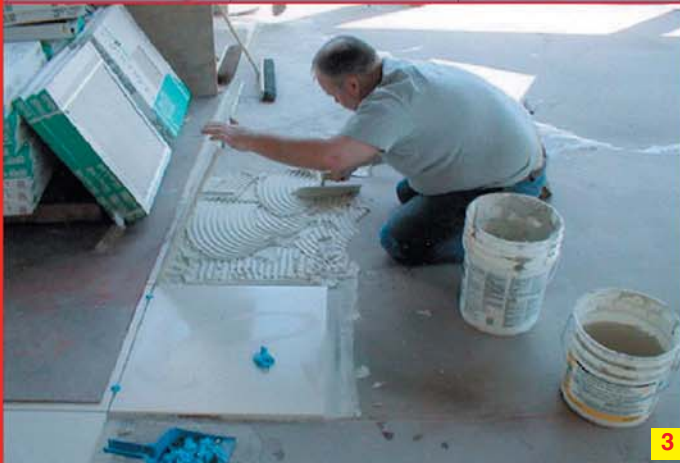
Photo 2. Tiles being installed in the showroom.
