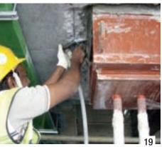
Rusting reinforcing rods needed to be treated since rusting formations on rods would have lead to concrete damage. MAPEFER corrosion-inhibiting cement mortar was chosen to prevent corrosion and rusting and to restore alkalinity. Before application, the rods had to be cleaned; thereafter, two coats of MAPEFER were applied with a brush.
