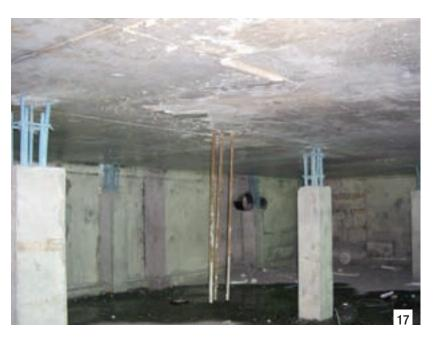
After the water seepage problem was curbed. ADESILEX PG2 SP and EPOJET LV were then applied onto as in the case of dry cracks.
