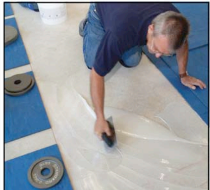
Ultrabond G21 polyurethane-based adhesive was used to install large-format rubber tile in MAPEI's employee gym.
