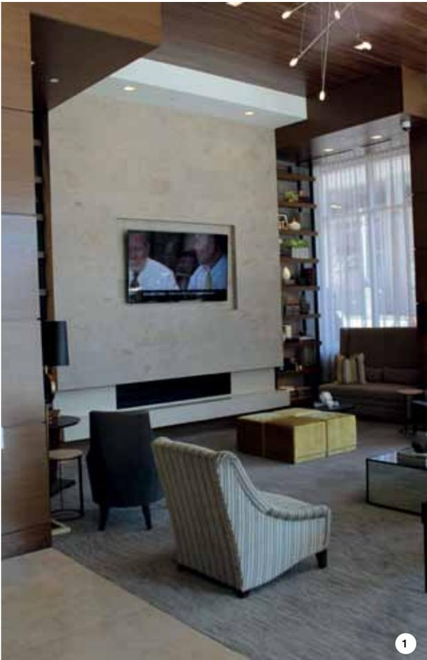
**PHOTO 1.** The installers cut the tile surrounding the fireplace down to 22,9 x 91 cm to create a beautiful floor-to-ceiling backdrop for the lobby. In these areas, they used ULTRAFLEX LFT for bonding ceramic tiles and ULTRACOLOR PLUS for grouting joints.
