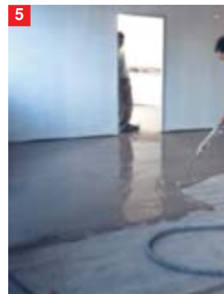
Photo 4. Levelling of the gaps and of the deeper joints with Nivorapid FF.
