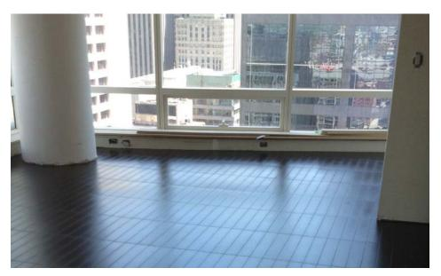
MAPEI began work on this project early in the planning stages. The original specification called for the use of a double-glue-down with cork to be used for sound reduction and then an adhesive. MAPEI offered a system warranty using Novoplan 2 to meet the substrate tolerances for engineered wood and Ultrabond ECO 995 as a one-step acoustical membrane and adhesive. MAPEI representatives made an initial presentation to Westbank Development.
