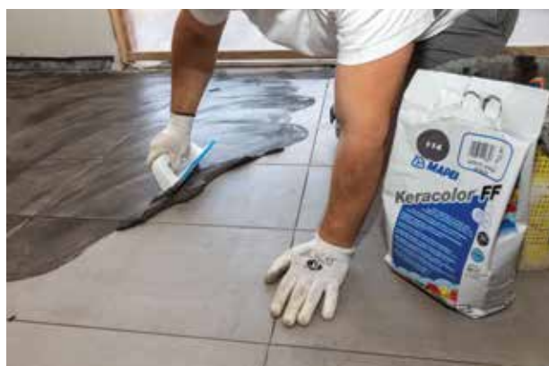
Ceramic tiles were bonded on the interior floors with KERABOND PLUS adhesive. ULTRACOLOR PLUS and KERACOLOR FF high-performance mortars were used to grout the joints.
