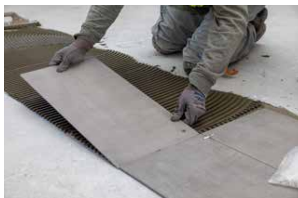
Ceramic tiles were bonded on the interior floors with KERABOND PLUS adhesive. ULTRACOLOR PLUS and KERACOLOR FF high-performance mortars were used to grout the joints.
