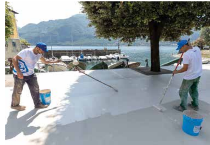
New, durable, resistant and safe surfaces were created by using MAPECOAT TNS EXTREME coloured epoxy-acrylic resin.
