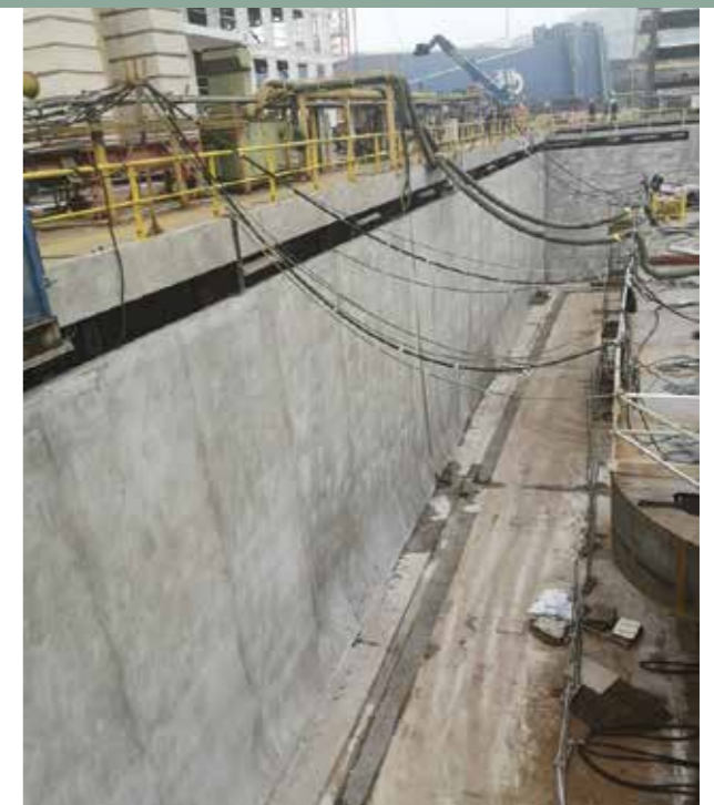
IN THE FACING PAGE. A view of the Fincantieri shipyard in Marghera, near Venice. ABOVE. Reinforcing rods were protected with MAPEFER anti-corrosion mortar (left), while several Mapei solutions were used to waterproof and repair the dock walls (right).
