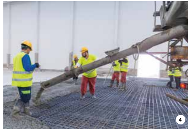
1. MAPEFER 1K, one-component, corrosion-inhibiting cementitious mortar, was used to protect reinforcement rods. 2. MAPEGROUT SV T and MAPEGROUT EASY FLOW were used to repair several areas of the concrete pillars. 3. After concrete was repaired, the surfaces were protected against carbonation by applying a coat of ELASTOCOLOR PAINT crack-resistant, elastomeric coating. 4. A new high performance concrete floor was completed with MAPECRETE SYSTEM.
