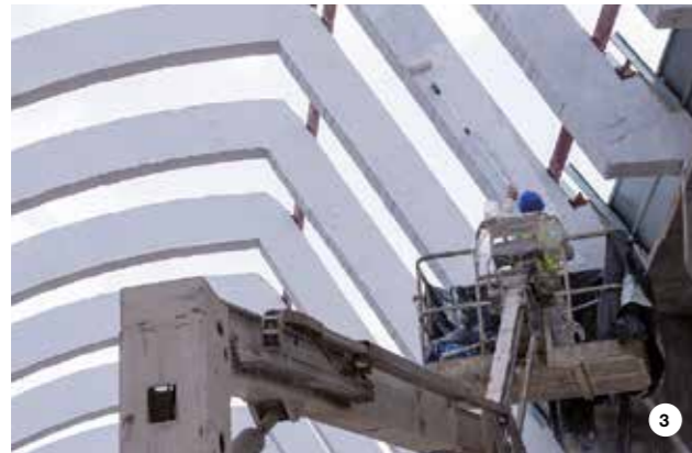
1. MAPEFER 1K, one-component, corrosion-inhibiting cementitious mortar, was used to protect reinforcement rods. 2. MAPEGROUT SV T and MAPEGROUT EASY FLOW were used to repair several areas of the concrete pillars. 3. After concrete was repaired, the surfaces were protected against carbonation by applying a coat of ELASTOCOLOR PAINT crack-resistant, elastomeric coating. 4. A new high performance concrete floor was completed with MAPECRETE SYSTEM.
