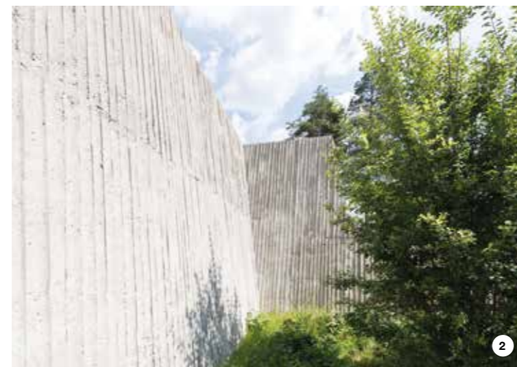
1. The Solothurn high school is an important example of the post-war "Brutalist" style of architecture and was lately renovated with Mapei solutions. 2. The pre-cast concrete elements used for the façade were repaired with MAPEGROUT THIXOTROPIC before protecting them with MAPEFINISH HD. 3. The damaged areas of the external stairs were repaired with MAPEGROUT 430 mixed with PLANICRETE after filling the cracks with EPORIP.
