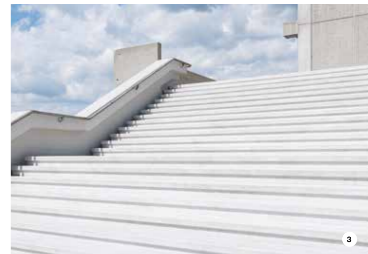
1. The Solothurn high school is an important example of the post-war "Brutalist" style of architecture and was lately renovated with Mapei solutions. 2. The pre-cast concrete elements used for the façade were repaired with MAPEGROUT THIXOTROPIC before protecting them with MAPEFINISH HD. 3. The damaged areas of the external stairs were repaired with MAPEGROUT 430 mixed with PLANICRETE after filling the cracks with EPORIP.
