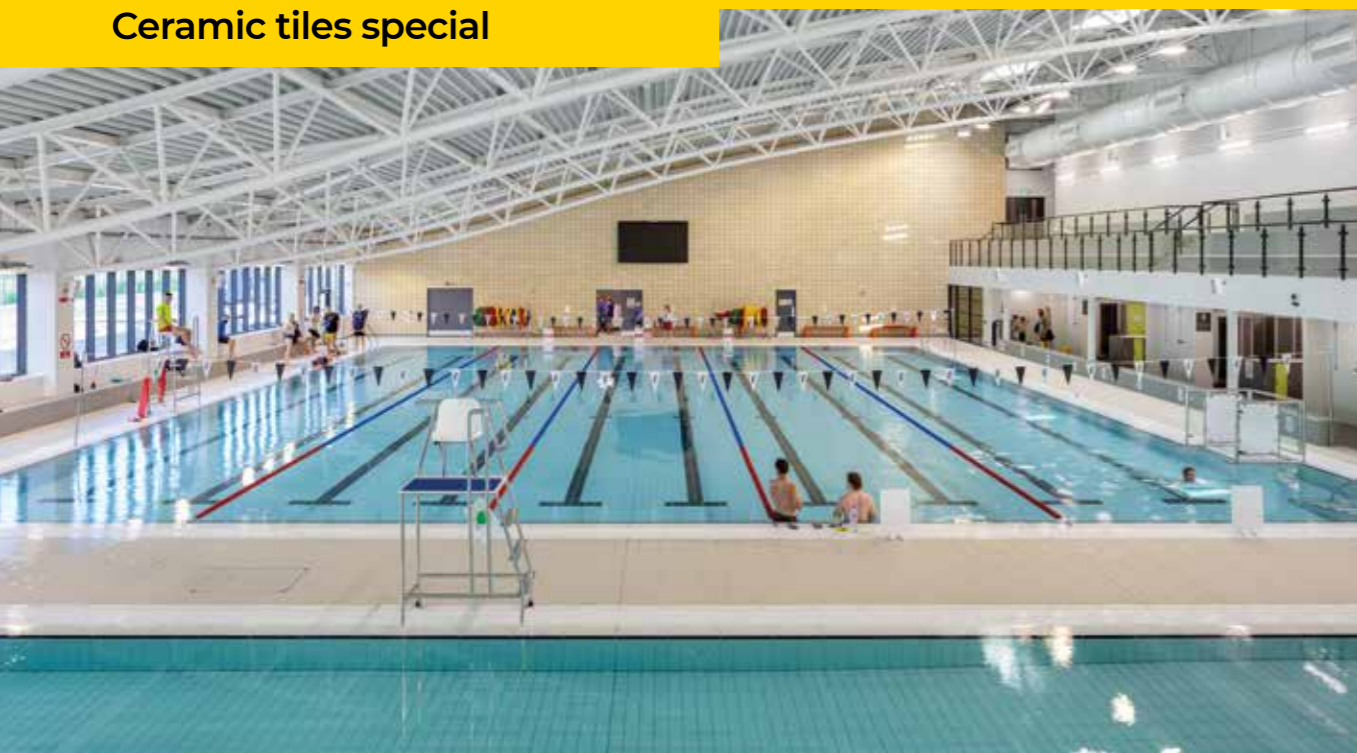
The ceramic tiles in the 10-lane pool were installed with KERAFLEX MAXI S1 and KERAQUICK S1*.
