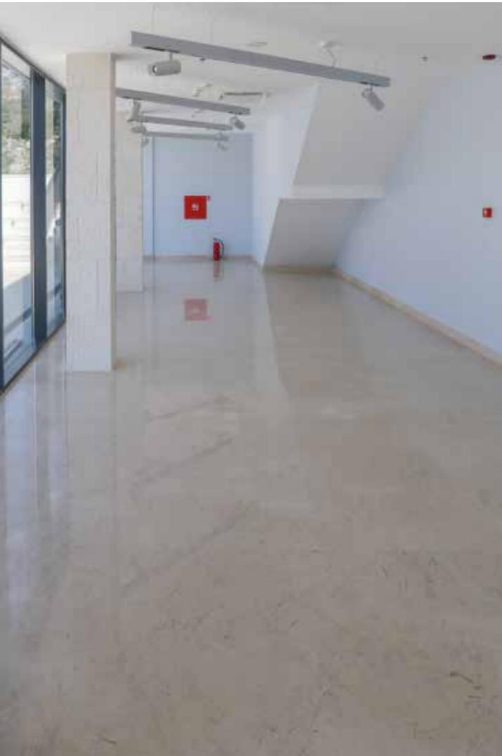
MAPEFLOOR SYSTEM 33, a self-levelling epoxy system, was used to create highly resistant resin floorings.
