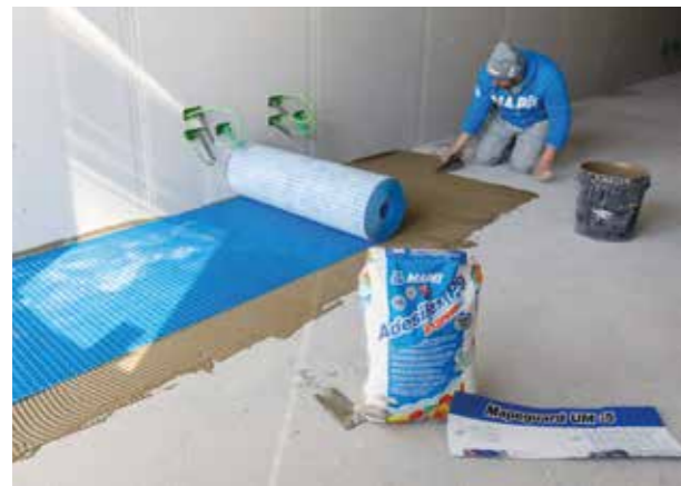
ABOVE, LEFT. MAPEGUARD UM 35 and MAPETEX SYSTEM anti-fracture membranes were bonded on the substrates in the corridors to ensure safe installation of ceramic tiles.
