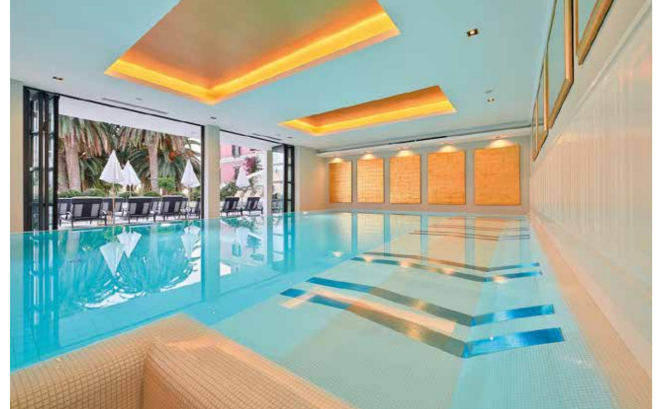
ABOVE. The substrates of the hotel's new swimming pool were levelled off with PLANITOP FAST 330 and the joints of the mosaic covering were grouted with KERAPOXY DESIGN epoxy mortar (later superseded by KERAPOXY EASY DESIGN).
