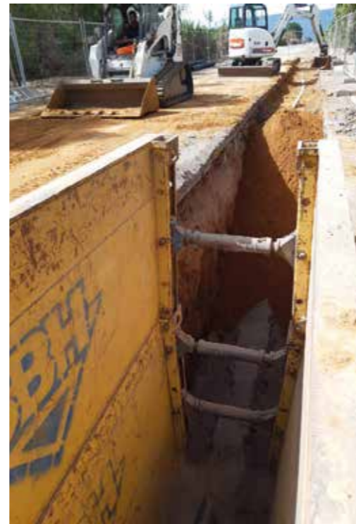
ABOVE. Excavating works for installing the sewer system.
