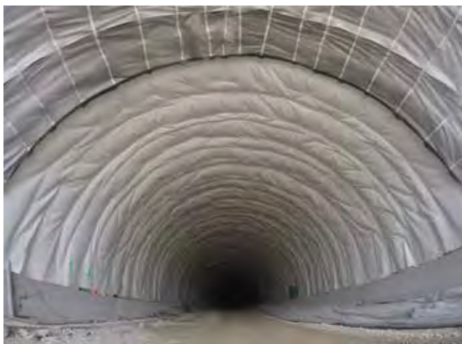
TOP OF THE PAGE. Applying shotcrete in the tunnels. BELOW, LEFT. Waterproofing the tunnels with MAPEPLAN TU S. RIGHT. The tunnel surfaces were painted with MAPECOAT W HRI epoxy coating.
