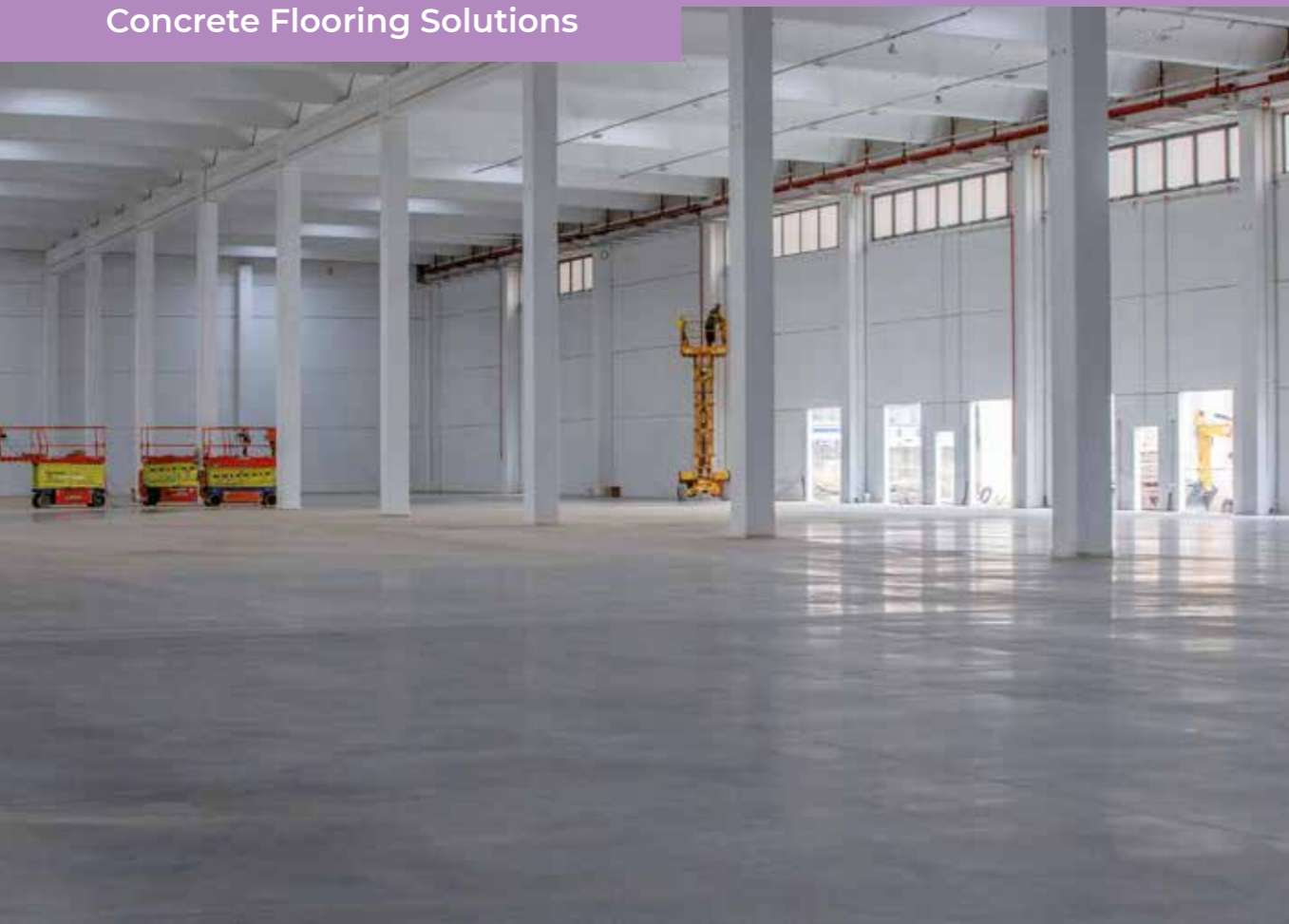
ABOVE. MAPECRETE LI HARDENER was chosen to finish off the floor, a surface treatment product in liquid form.
