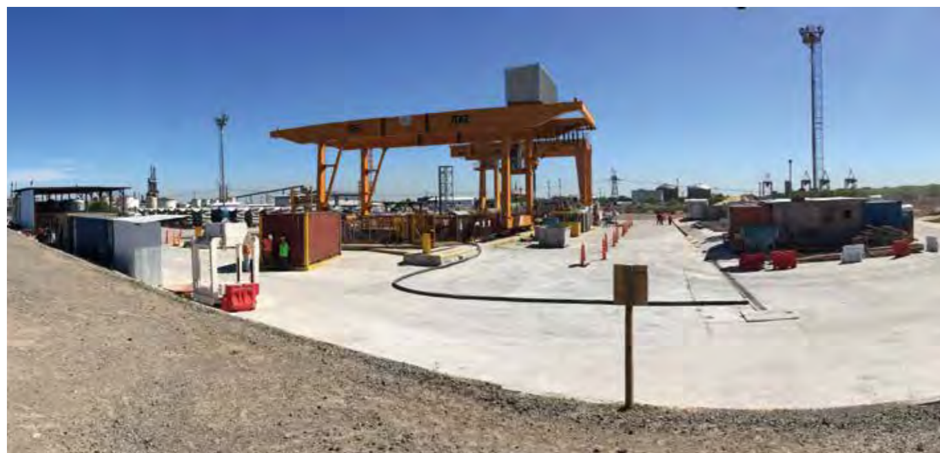
View of an external section of the Matanza-Riachuelo Basin Lot 3.
