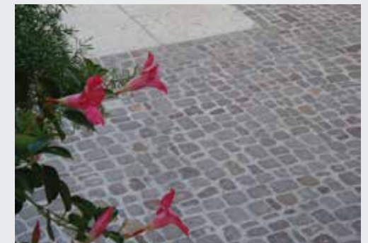
Cobbles and cubes in various sizes were installed in a characteristic pattern and grouted with MAPESTONE PFS2 to make it easier for pedestrians to walk cross.
