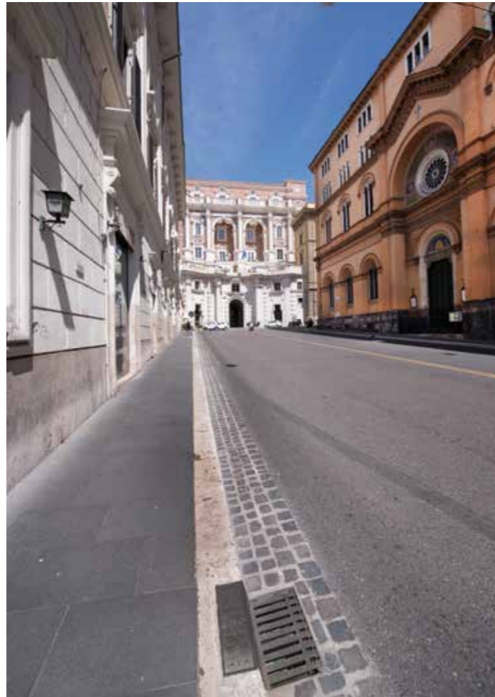
ABOVE. Apart from being firmly embedded right up to the edge of the paving, the gutters were installed in such a way that they provided a sound housing for the drain covers for the rainwater to flow into.
