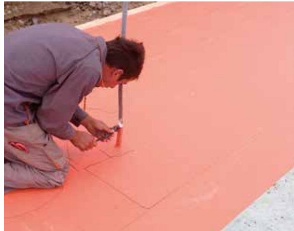
ABOVE. MAPEPLAN UG waterproofing membrane was used to waterproof the foundations.
