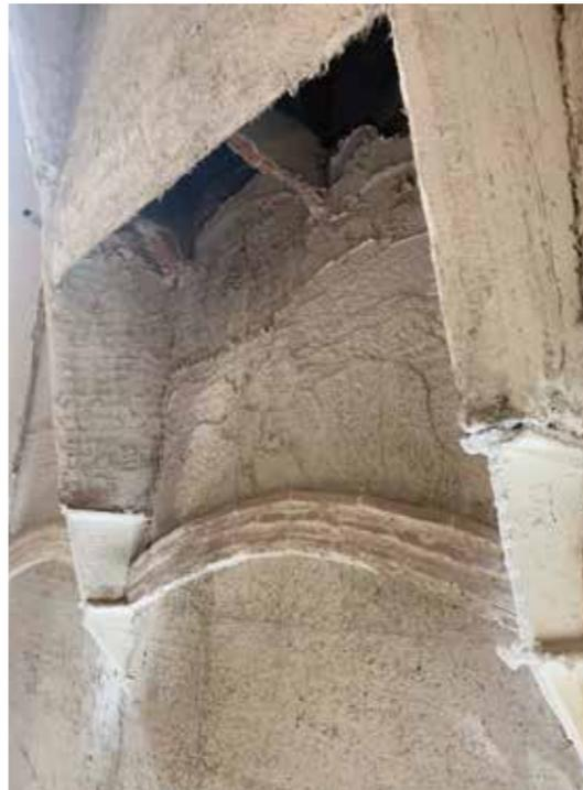
Work started with the application of a first coat of PLANITOP HDM RESTAURO two-component, pre-blended, fibre-reinforced, high ductility mortar made from natural hydraulic lime (NHL) and Eco-Pozzolan to level off the substrate. MAPEGRID G 220 alkali-resistant glass fibre mesh was then placed on the mortar, a product which is particularly recommended for “reinforced” structural strengthening work on stone, brick, tuff and mixed masonry structures.
