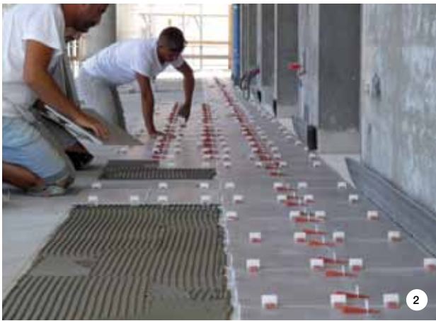
In the interiors, after building the screeds with TOPCEM PRONTO, the porcelain tiles were installed with KERAFLEX MAXI S1 cementitious adhesives. Joints were grouted with ULTRACOLOR PLUS high performance mortar, both in interiors and exteriors.
