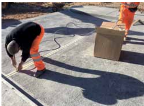
Sealant applied along the lanes of the toll stations
