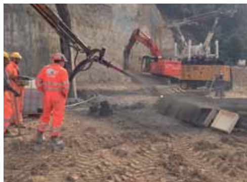
Trials of the shotcrete in the Sant'Urbano tunnel
