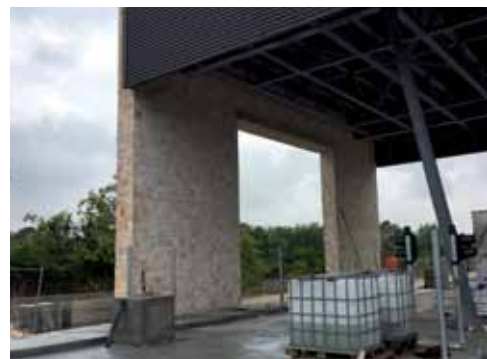
Installation of the stone covering on the toll stations
