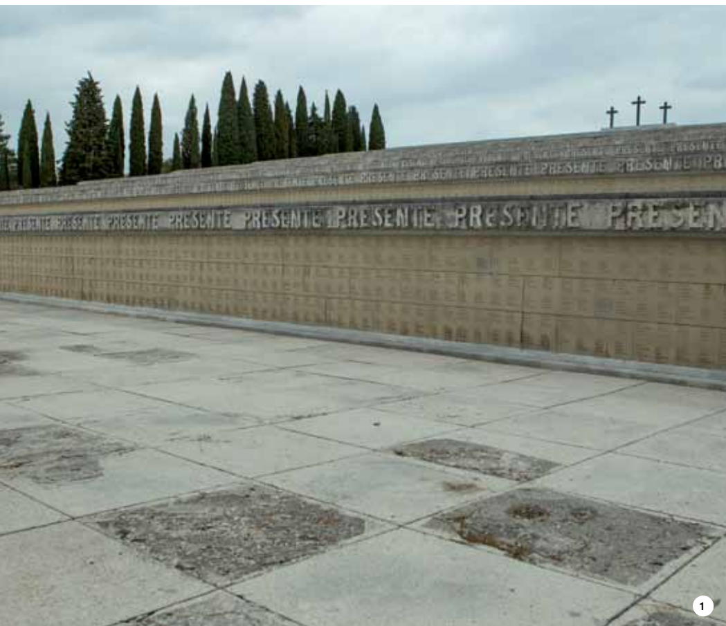
PHOTO 1. The damaged slabs on the piazza before restoration works.
