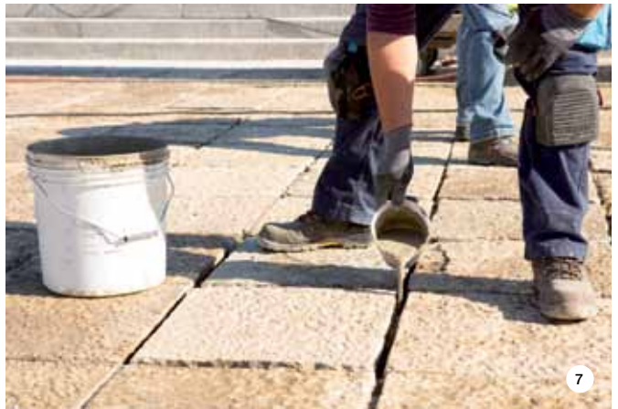
PHOTO 4. MAPEWASH PO set retardant was applied on the substrate.
