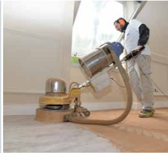
The substrates were sanded around one hour after applying ULTRACOAT BINDER, which is mixed with sawdust. The surfaces were then finished with ULTRACOAT HIGH TRAFFIC varnish.
