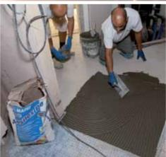
All the substrates in the kitchens were waterproofed with MAPELASTIC TURBO two-component, flexible cementitious mortars before bonding the 30x60 cm porcelain tiles with KERAFLEX MAXI S1. In the underground service area 20X20 cm ceramic tiles were, on the other hand, installed with ADESILEX P9.
