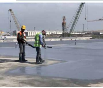
tive and negative water pressure. Prior to the application of MAPELASTIC FOUNDATION, PRIMER 3296 acrylic primer with strong penetrating action had been applied to level off the surface and improve its bonding properties.
