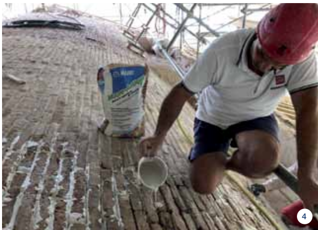
PHOTO 3. The FRP SYSTEM was used to strengthen the apse.
