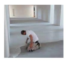
multipurpose, neutral-coloured epoxy formulate with excellent resistance to chemical agents and abrasion, mixed with white MAPECOLOR PASTE coloured paste and DYNASTONE TZ, 8 mm thick aggregates.
