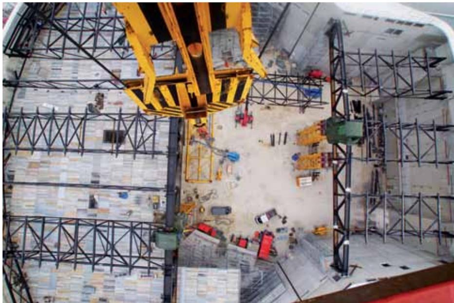
**ABOVE.** MAPEFILL F mortar was used to anchor metal and concrete elements.
