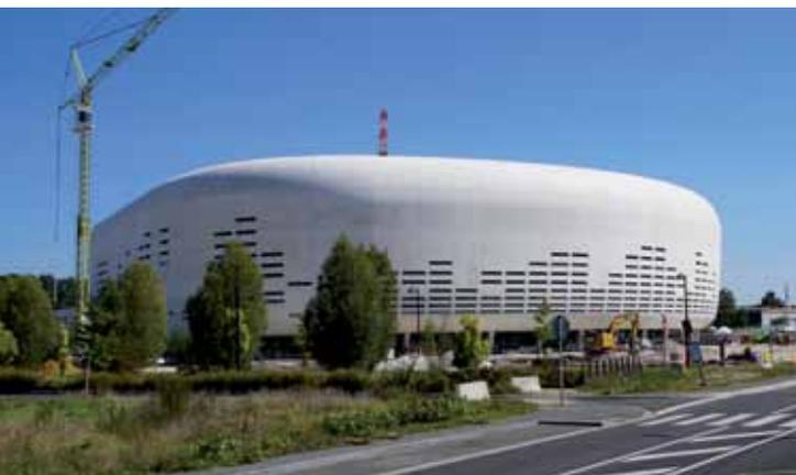
**ABOVE.** NIVOPATE Fin smoothing compound was used for the finishing of the external concrete shell.
