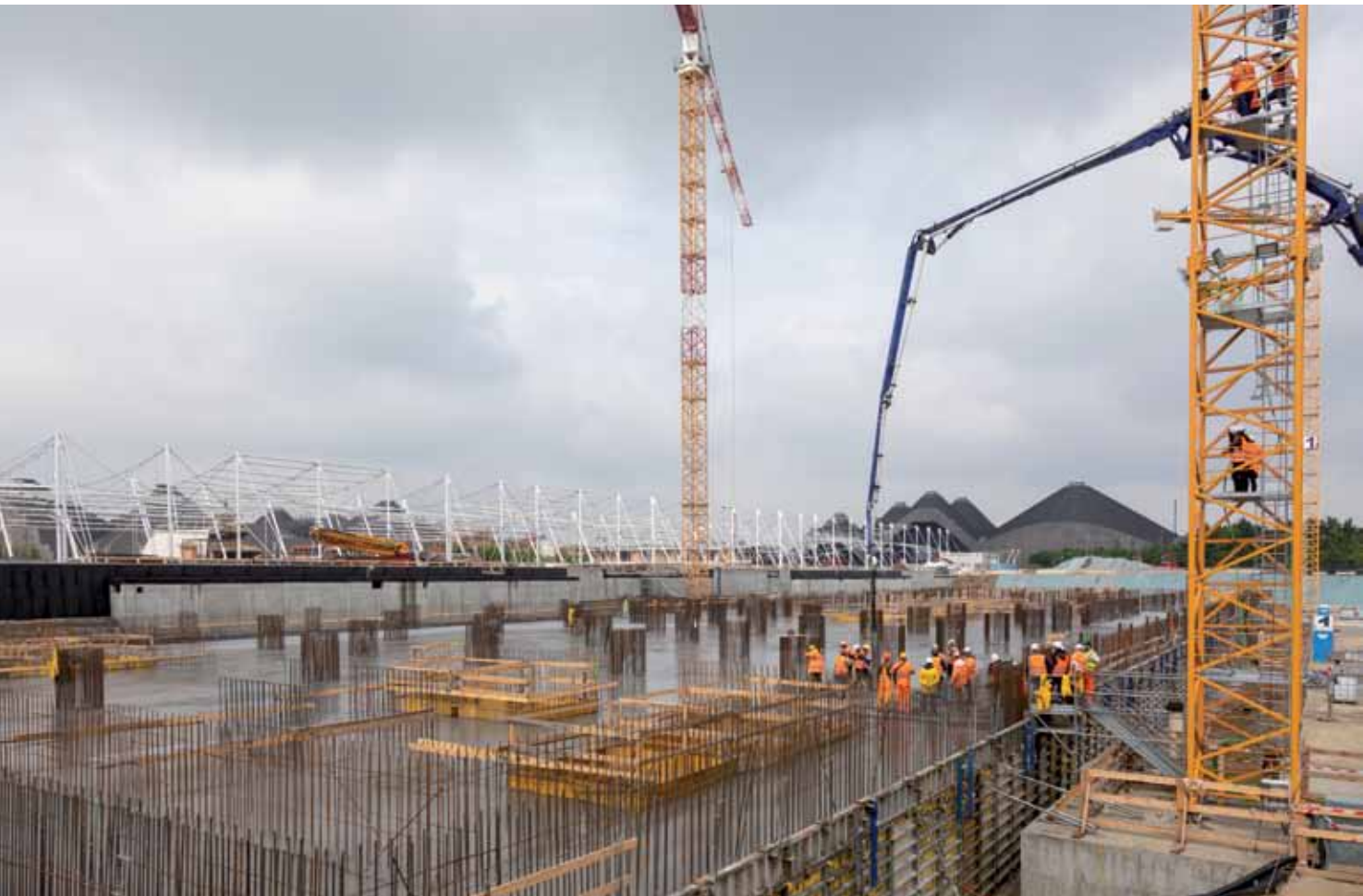
33,000 m 3 of concrete were pumped non-stop for 94 hours last May to build the foundation slab of the hospital.
