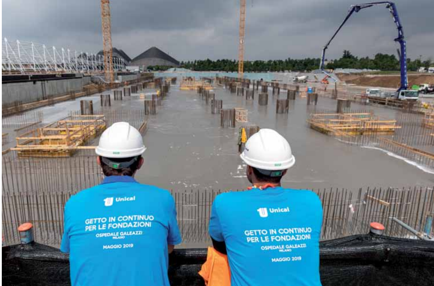
A special, bespoke concrete was designed for the pour. The new Galeazzi Orthopaedics Institute is being constructed in the former Expo area in Milan.
