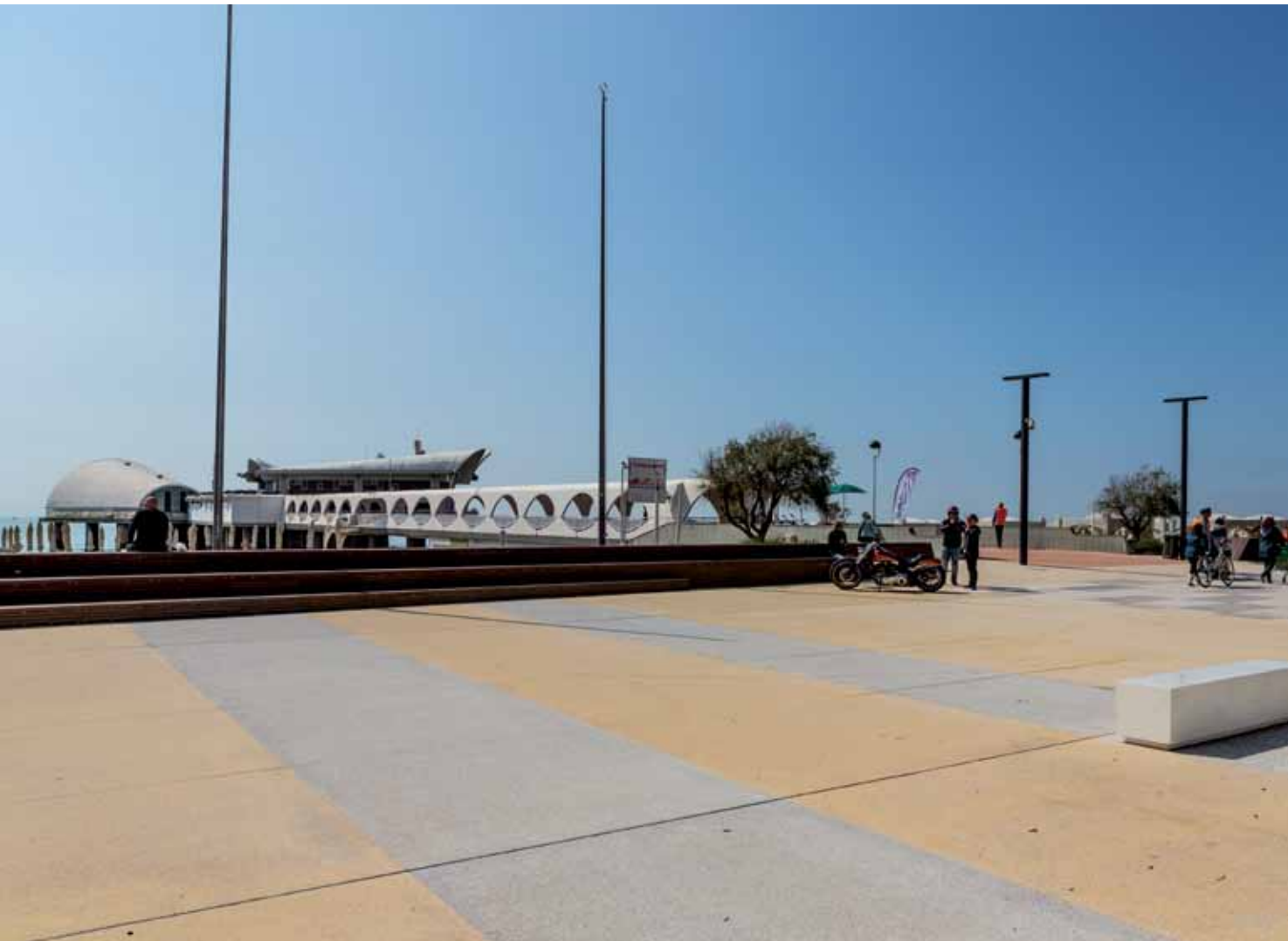
Along the Trieste waterfront in Lignano stone paving was installed with the MAPESTONE system while the exposed aggregate concrete paving was built using the MAPEI COLOR PAVING® system.
