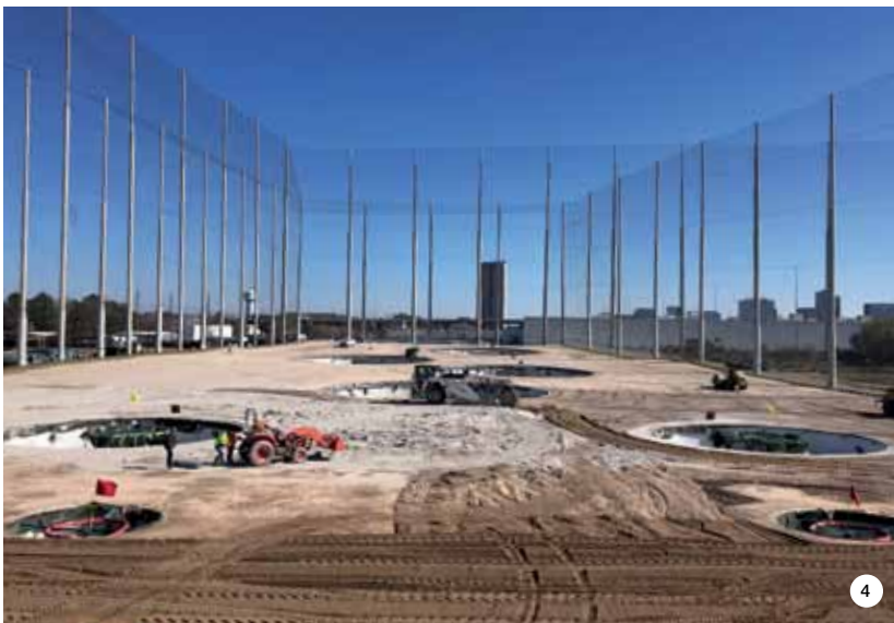
Stabilisation of the practice area with MAPESOIL 100 (notice the height of the fences).
