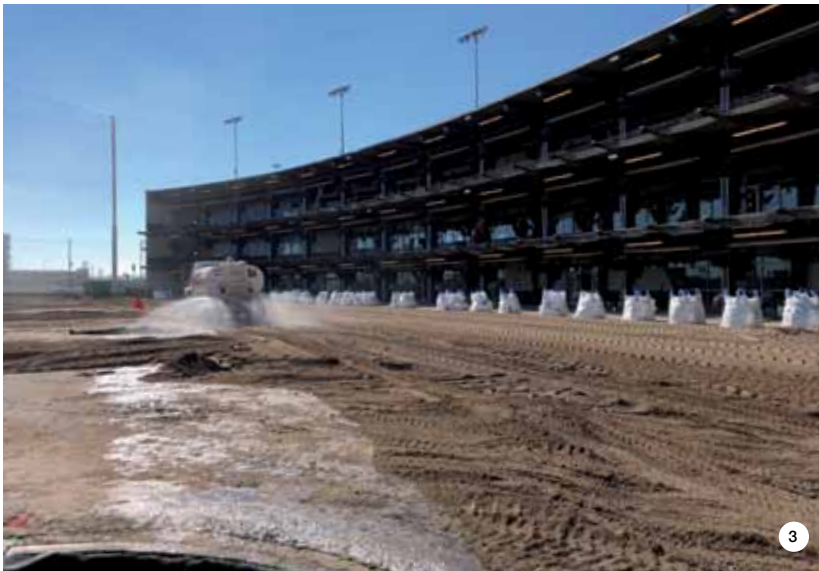
Preparation of the area to be treated with MAPESOIL 100.
