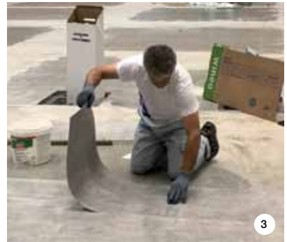
1. Before installing the floors, the substrates were skimmed with PLANIPREP FAST TRACK. Flatness was restored to the substrate where required by using NIVORAPID and LATEX PLUS. 2, 3, 4. PURLINE organic flooring by Wineo was installed with ADESILEX G20 adhesive. 5. ULTRABOND MS RAPID rapid-setting assembly adhesive and MAPESIL AC sealant were used to seal the manholes.
