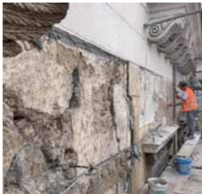
ABOVE. The palace after completion of the works. LEFT. After removing the detached masonry and renders and cleaning the substrates, the façades were painted and protected with SILANCOLOR BASE COAT and SILANCOLOR PAINT PLUS.
