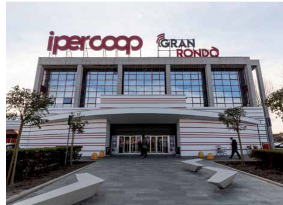
LEFT. A view of the external arcade upon completion of the restyling work. RIGHT. An external view of the shopping centre.
