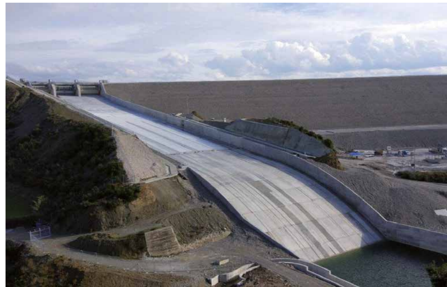
ABOVE. MAPEFLEX PU65 was used to seal joints in the concrete elements used for the spillway.
