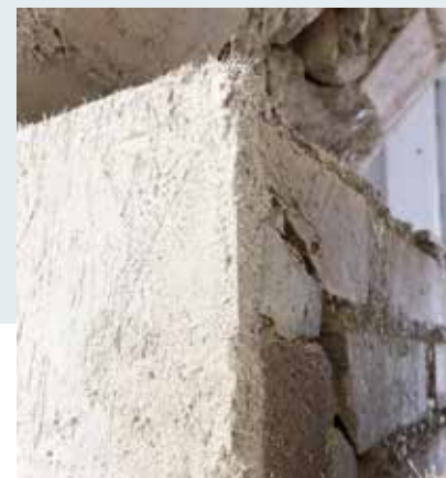
Close-up of the product applied (left) and the masonry panel after completing the strengthening work (right).
