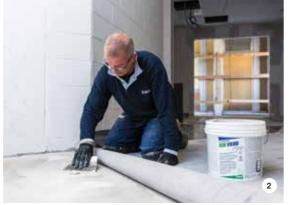
1. The floor substrates were levelled with ULTRAPLAN ECO before bonding rubber coverings thereupon.
