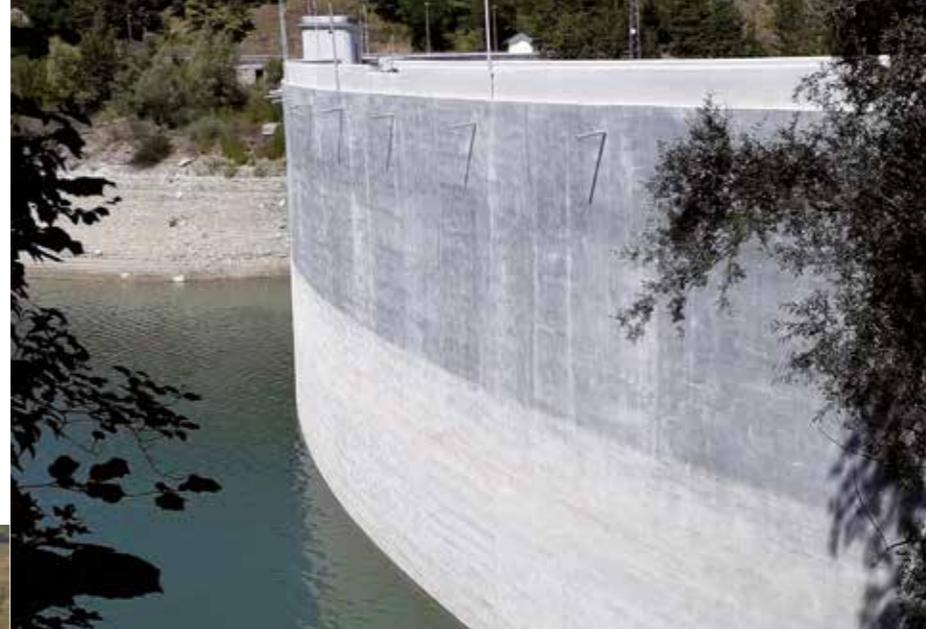
**LEFT.** The lake-side concrete wall was repaired by applying MAPEGROUT EASY FLOW, sulphate-resistant, fibre-reinforced, shrinkage-compensated, thixotropic mortar.
