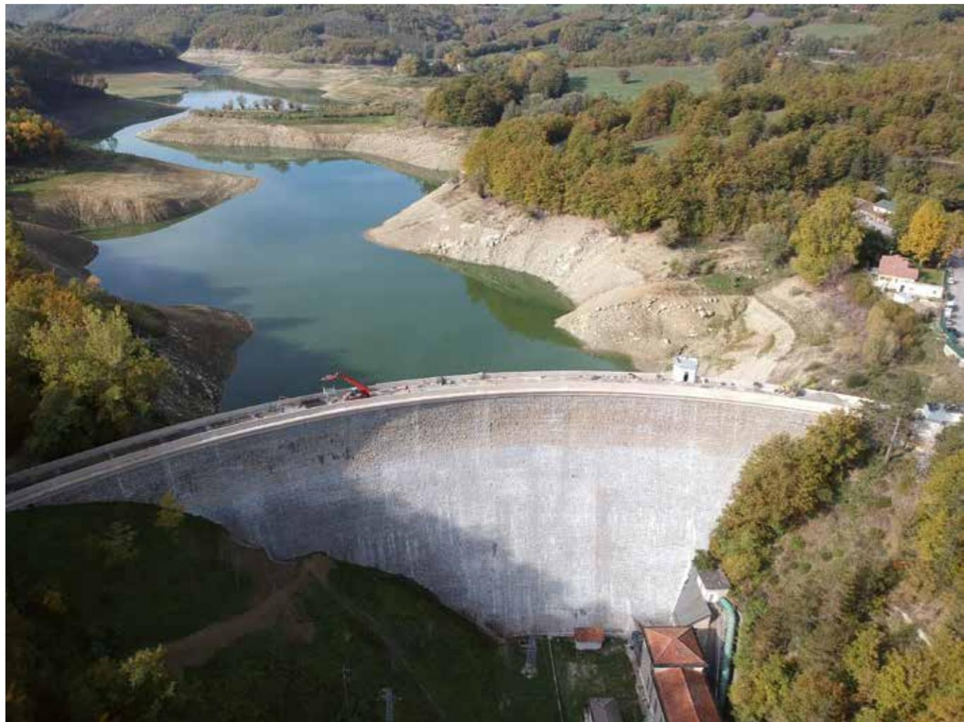
Construction of the reservoir at Scandarello near Amatrice (Province of Rieti, Italy) to produce and distribute electricity, commenced in 1918 following a decision by the Italian energy company U.N.E.S. which was acquired in 1962 by the energy group ENEL. The dam was designed by Angelo Omodeo in 1917 and is a concrete gravity-type structure which went into service in 1924. The Tronto lake, which covers an area of around 2 km<sup>2</sup> and is around 40 m deep, is fed
