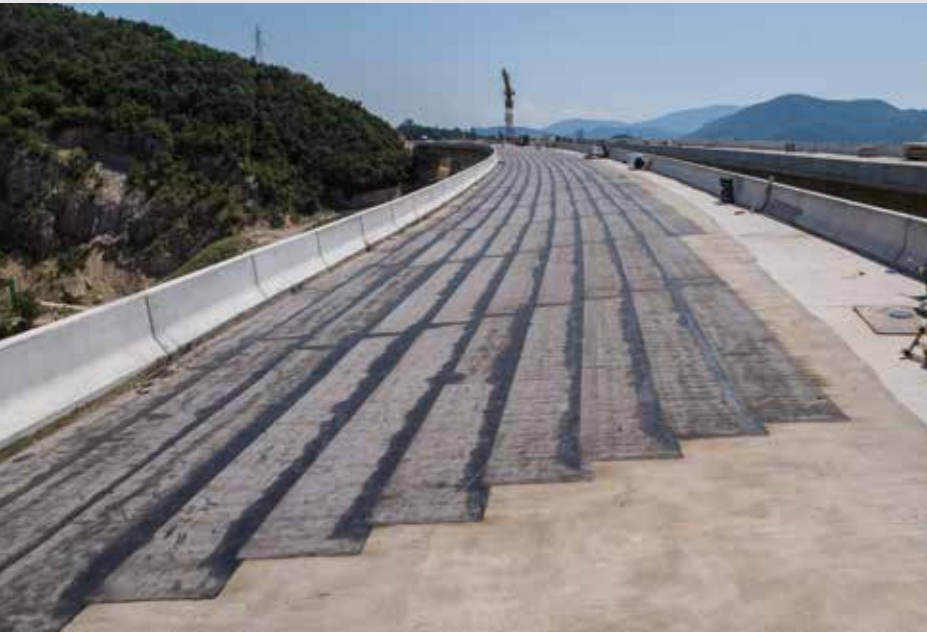
LEFT. Waterproofing the road surfaces with Polyglass solutions.
