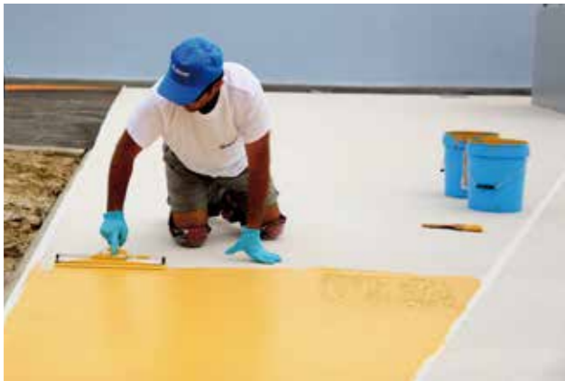
The 5-a-side football pitch was coated with MAPECOAT TNS MULTISPORT PROFESSIONAL, a multi-layered, acrylic resin-based system, which is used for creating polyfunctional sports surfaces with high resistance to wear, UV rays and atmospheric agents.
