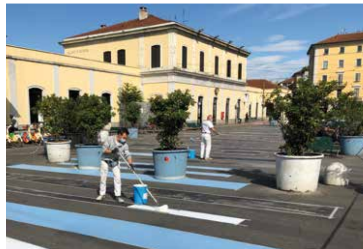
Two coats of MAPECOAT TNS EXTREME coloured epoxy-acrylic resin-based coating was applied on the surfaces of Piazzale Porta Genova. Work was completed by applying MAPECOAT TNS PROTECTION protective finish.
