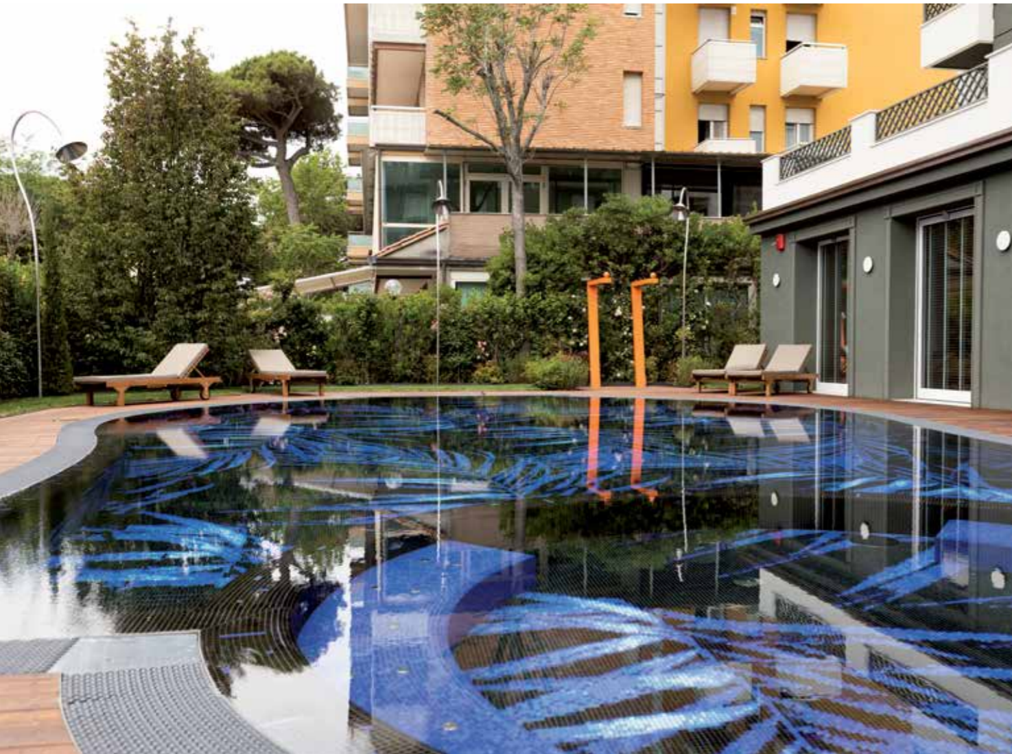
Mosaic tiles supplied by Mosaico+, a subsidiary of the Mapei Group, were bonded in the swimming pool with ULTRALITE S1 cementitious adhesive with no vertical slip.
