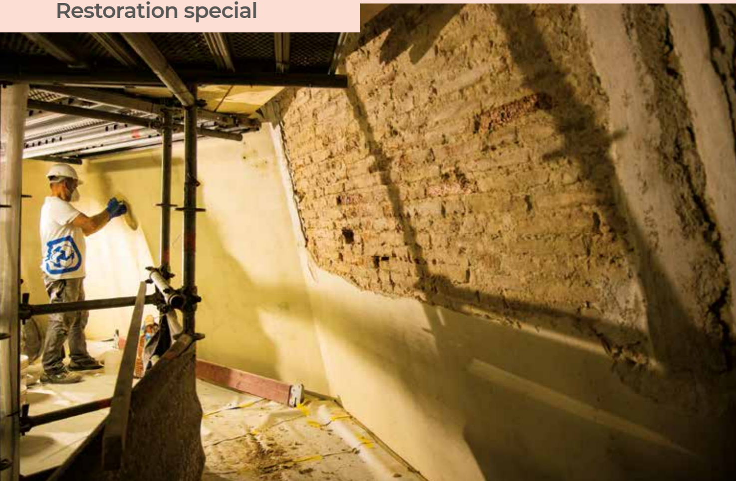
ABOVE. Portions of render detached from their substrates were consolidated and re-bonded by injecting MAPE-ANTIQUÉ F21.
