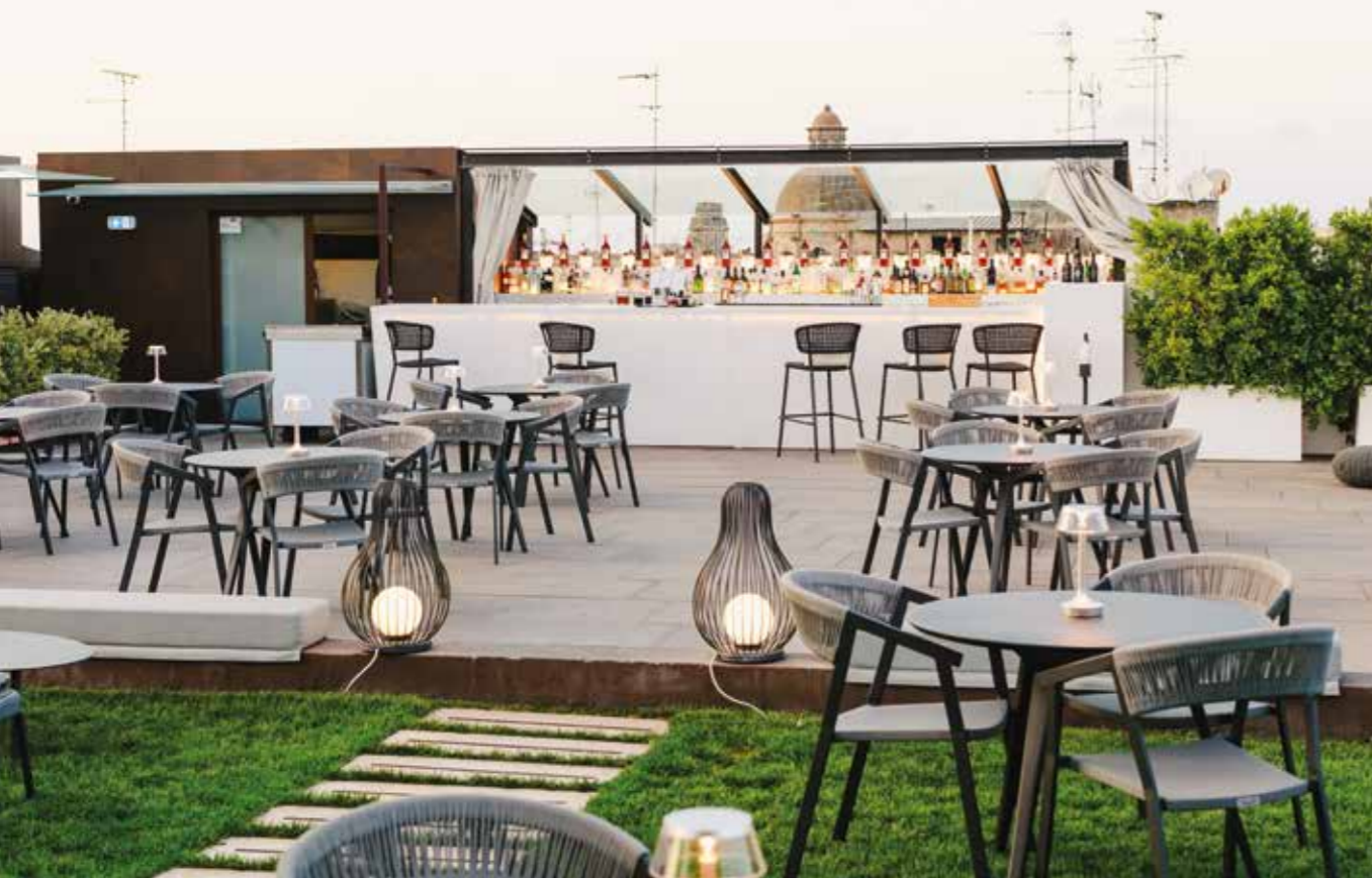
ABOVE. The substrates on the roof garden were waterproofed by applying PURTOP 1000 membrane.
