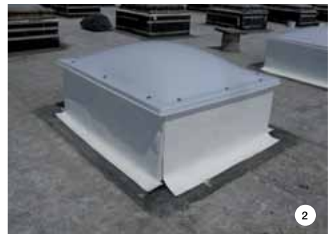
PHOTO 1. Condition of the roof prior to the upgrade.
