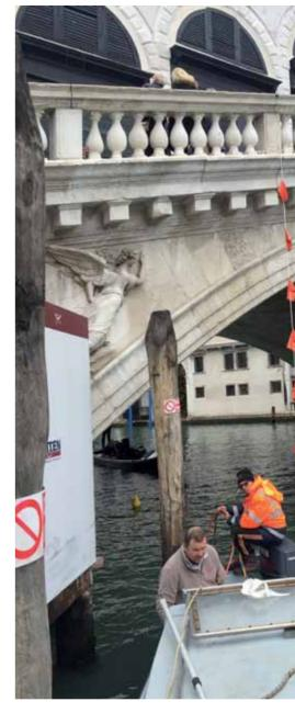
The joints between the stones immersed in the waters of Canal Grande were pointed by injecting STABILCEM very fluid expanding cementitious binder admixed with MAPEPLAST UW antiwashout powdered admixture that has been specifically developed for underwater concrete. In the areas of pavement that needed to be structurally strengthened, the stone slabs were bonded and sealed with ADESILEX PG2 two-component thixotropic epoxy adhesive for structural bonding.
